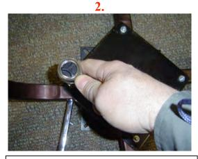
Remove the (4) 7/16" bolts and hex nuts that bolt through the bottom side of the swivel, top base plate, square tubular leg frame, and lower base plate.
